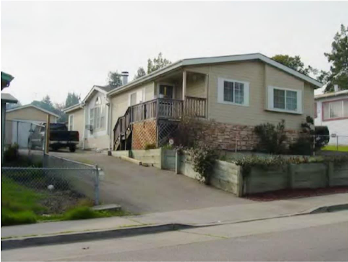
Figure 2.4: Two-section HUD-Code Home
