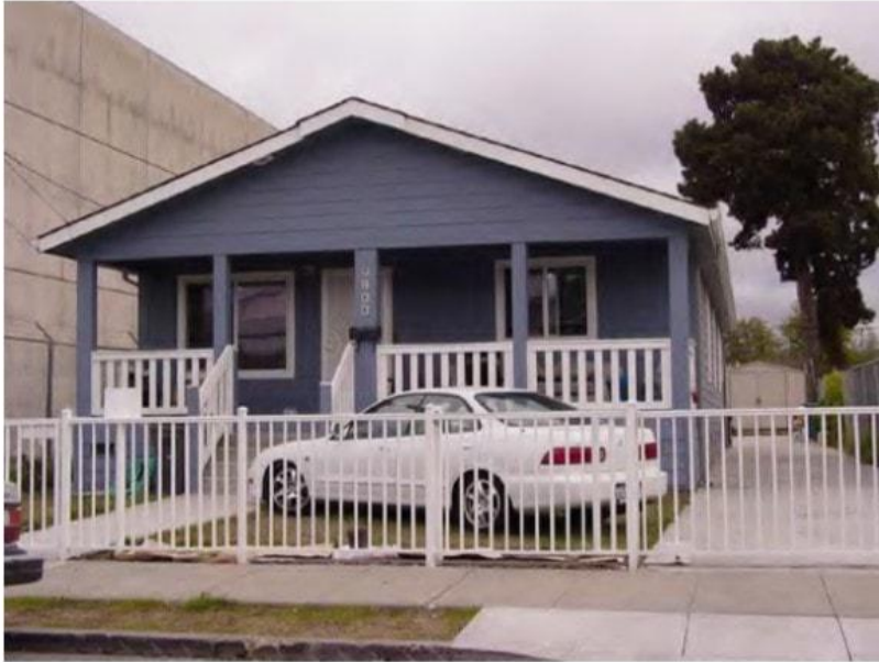
Figure 2.2: Multi-section Single-family Manufactured Home
