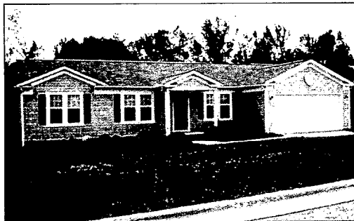
Mid-range double-section home with garage
