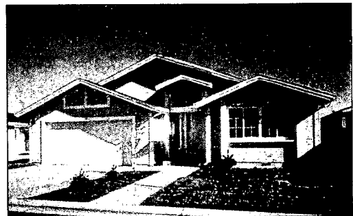
1990's multi-section home with site-built garage and roof section
