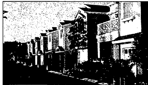
Row of 2-story units nearing completion in Orange County, California
