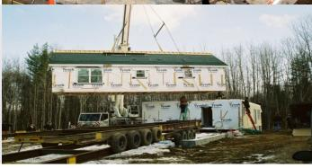
**Modular homes** are constructed using individual sections, called modules, built in a factory, and assembled on site. Modules can be of different types—fully enclosed modules, partially open-sided modules, or open-sided modules.
