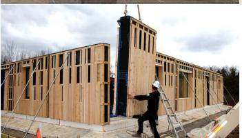
**Panelized homes** are made of standardized wall panels that can be assembled on site or in a factory off site. There are two general types of panels: open, which consist solely of framing, and closed, which include plumbing, insulation, and electric wiring.
