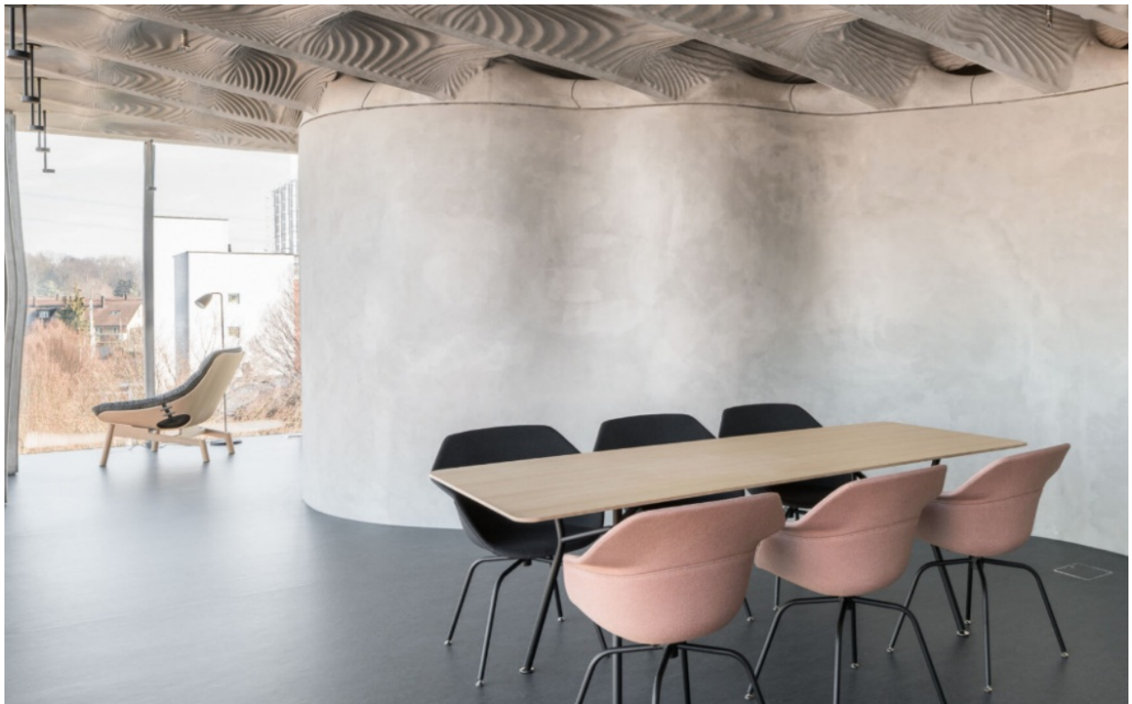
Interior view of the curved wall produced using a robot, or “fabricator”
