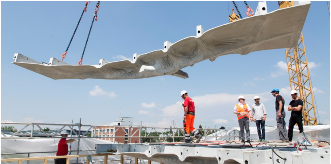
The "Smart Slab", used as the roof, is claimed to be the first concrete slab fabricated with a 3D-printed formwork
