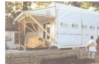
Manufactured home section installed on foundation (courtesy, MHI).
