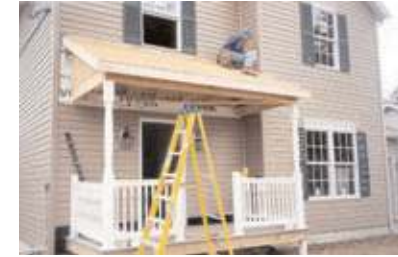
Finishing crew constructs site-built elements such as porches (courtesy, Unibilt Industries, Inc.).
