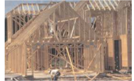
Traditional ‘stick-built’ construction (courtesy, SWA).
