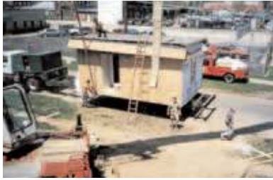
Modular housing arrives on the site as nearly finished modules (courtesy, MHI).
