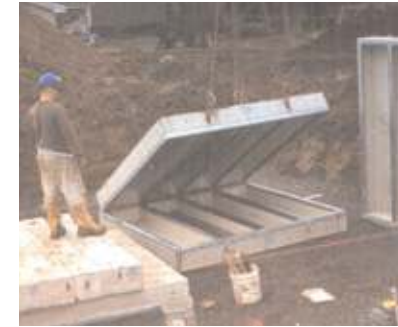
Precast concrete foundation systems (courtesy, SWA).
