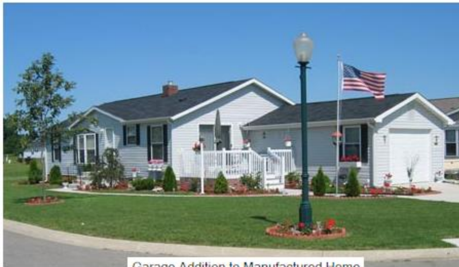
Garage Addition to Manufactured Home
